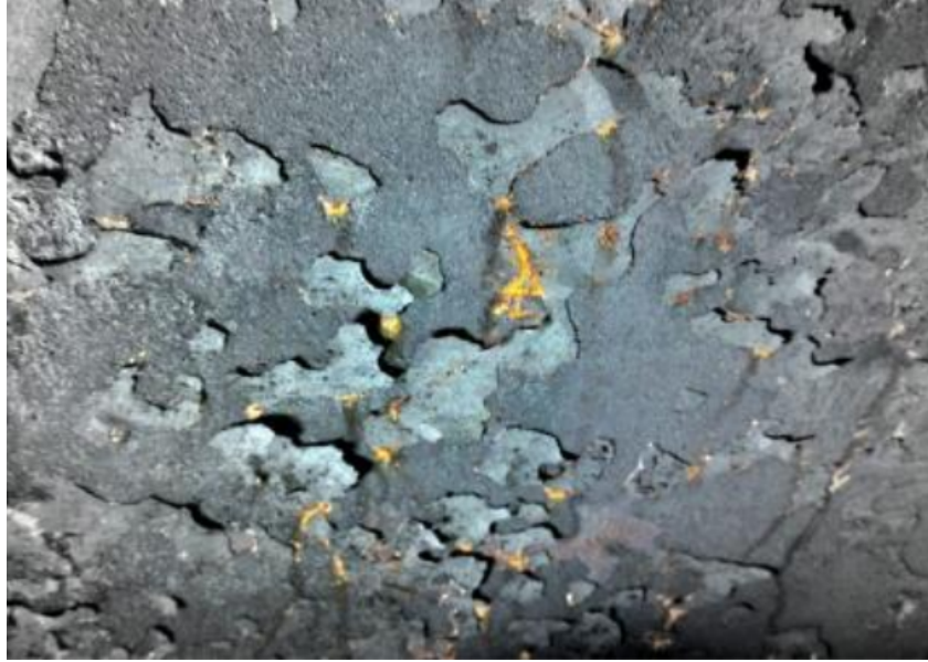
Figure 10. Diagram showing exfoliation corrosion [32]
