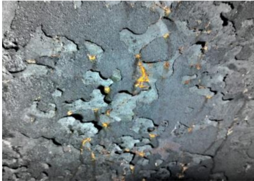
Figure 10. Diagram showing exfoliation corrosion [32]
