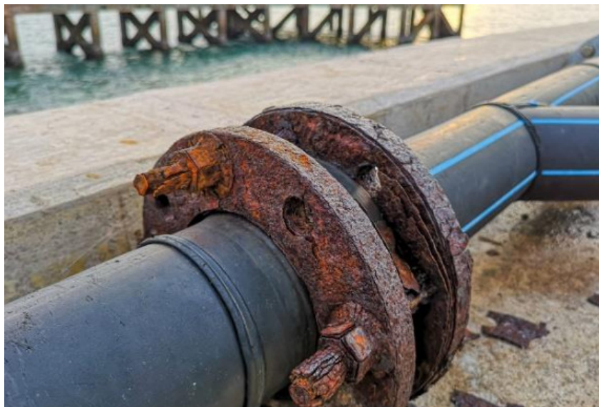
Figure 6. Diagram showing high-temperature corrosion [32]
